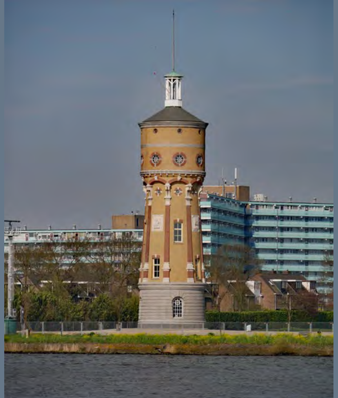
Dordrecht Water Tower
