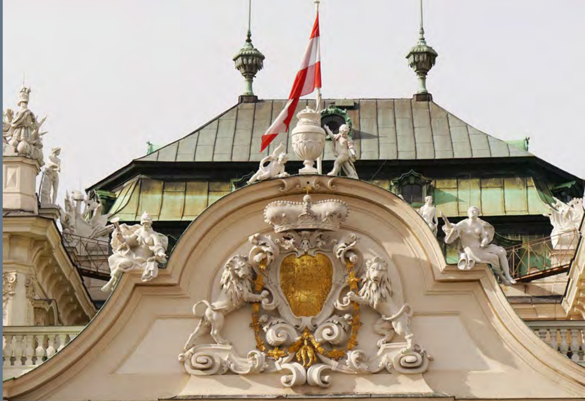
Upper Belvedere Palace Roof Detail
